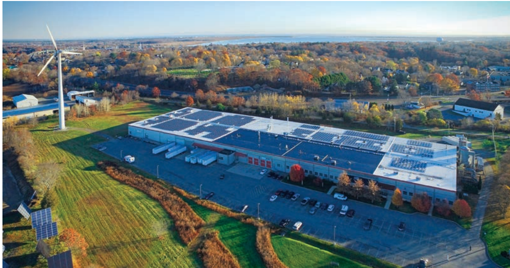
The Mark Richey Woodworking/WallGoldfinger Furniture, Newburyport, Mass., factory, is powered by on-site solar and wind.
